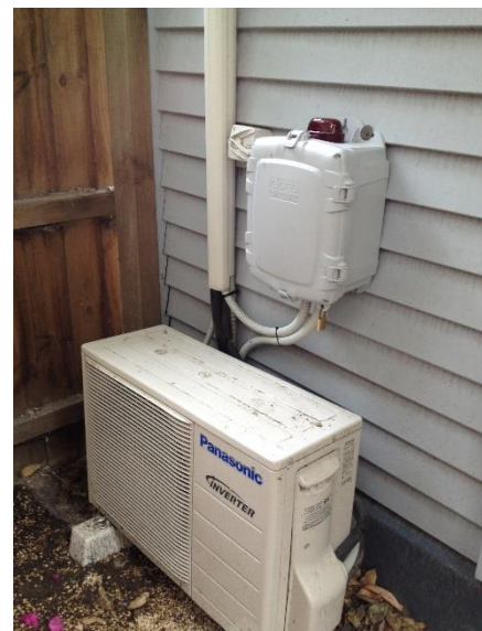
Typical Alarm Panel Installation
